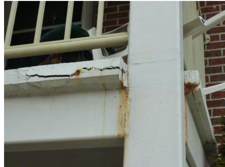
Typical failing concrete at rusting steel reinforcing and connections.
