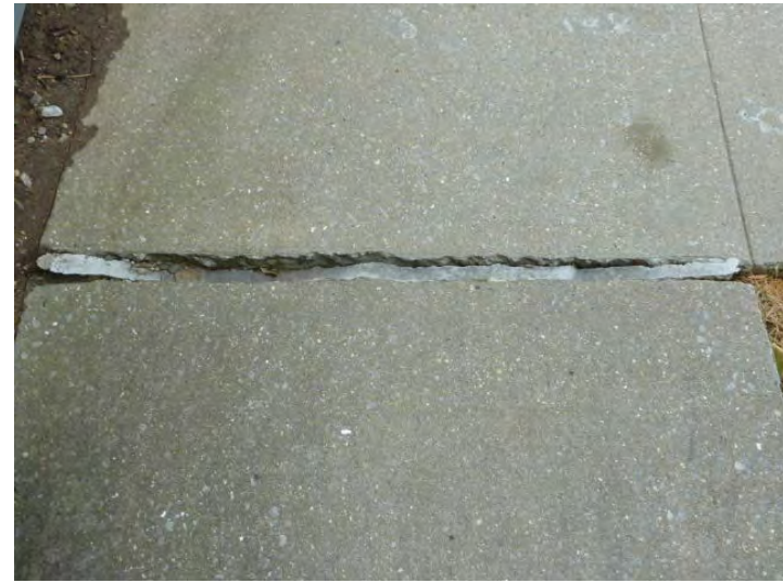
Typical failed joint in concrete walks site-wide.
