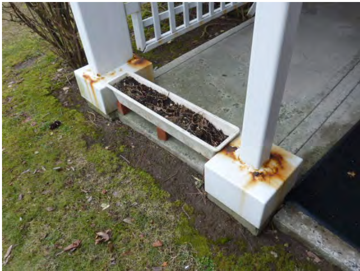
Typical rusting at steel tube column bases.
