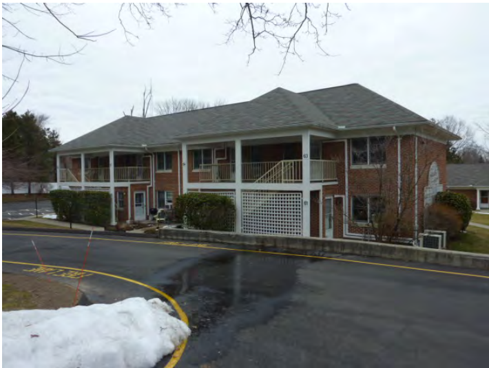
Typical front elevation with roofs over open egress stairs, second floor porches and ground floor patios. Asphalt paving and striping is new site-wide.
