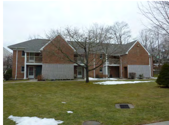
Typical rear elevation with egress stair towers and second floor porches and ground floor patios.
