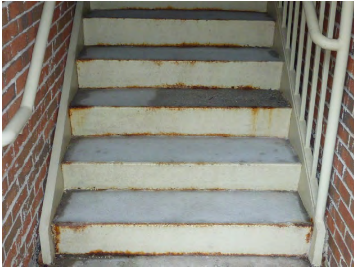
Typical rusted steel pans at stairs.
