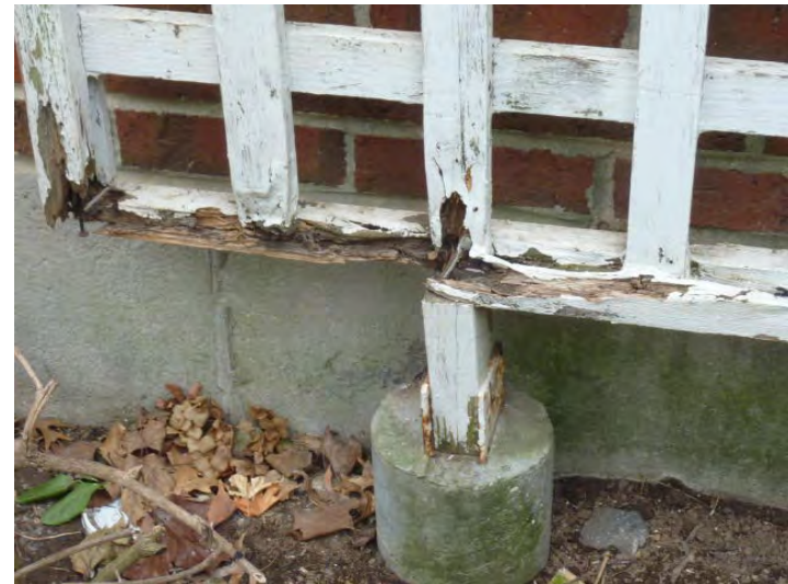
Typical rotted wood trellis site-wide.
